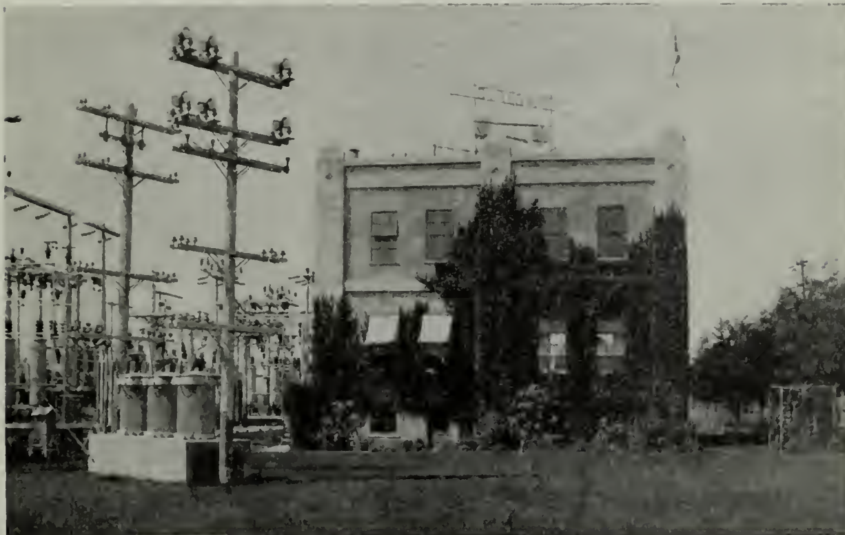
Posco Substation - constructed in 1918 by Pacific Power & Light Company.
